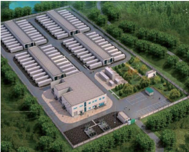
◎ Anhui Jinzhai Independent Energy Storage Power Station Project
