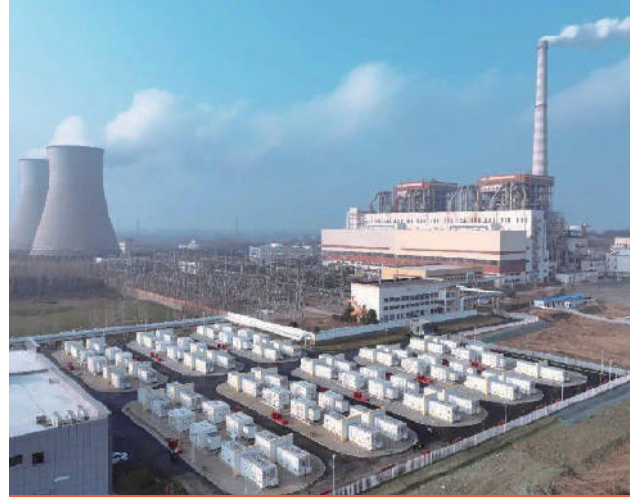
◎ Huaibei Wanneng Energy Storage Power Station Project
